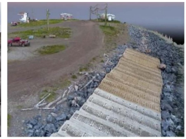
(c) Revetment using articulated concrete mats (Tuktoyaktuk, N.W.T.)
