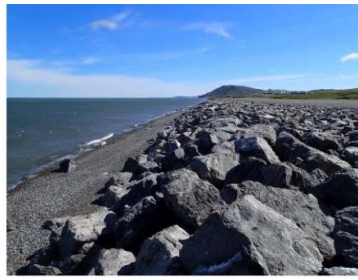
(a) Rock revetment (Cape Lisburne, Alaska)
