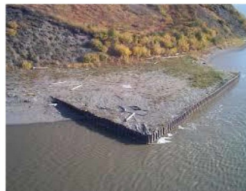
(e) Bulkhead using sheet-piles (Tununuk Point, N.W.T.)
