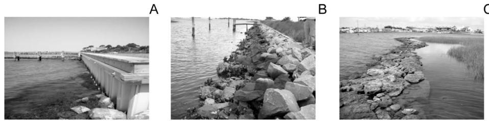
Fig. 1. Photographs of shoreline types: A) a bulkhead: a vertical structure typically constructed of vinyl composite, concrete, asbestos, or treated wood placed at or above the observed high water mark; B) a riprap revetment: a sloped structure typically constructed of granite, marl, or concrete placed at or above OHWM; and C) a sill: a structure typically constructed of granite, marl, or oyster shell, seaward of marsh.
